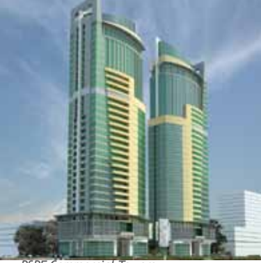
PSPF Commercial Towers
