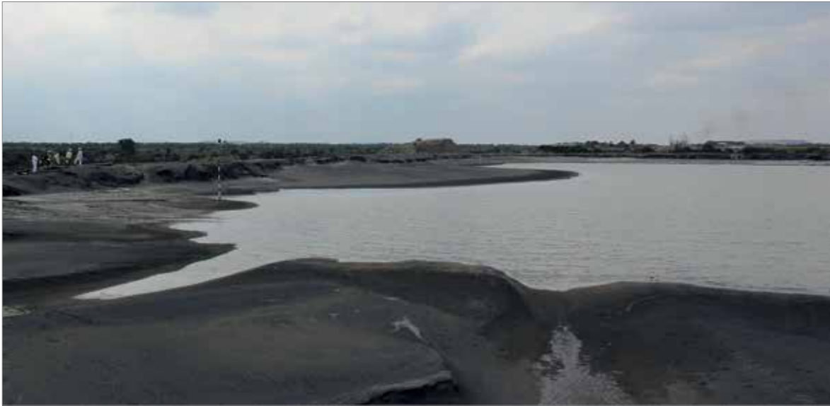
Fig. 5.8: Mooinooi tailings dam, 25 km east of Rustenburg, with an average height of 6 m (photo: DERA 2014).
