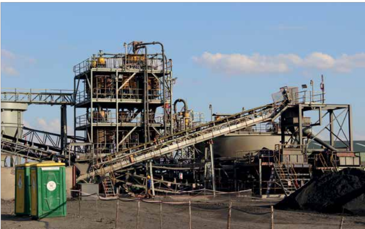
Fig. 3.16: Beneficiation plant at Thaba Mine (photo: DERA 2014).
